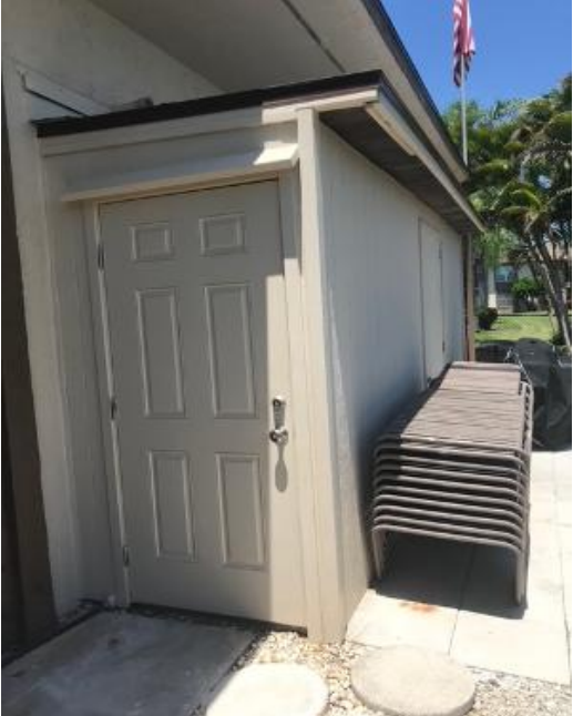
The new, improved storage enclosure
