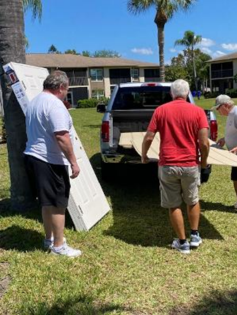
Unloading materials for the enclosure
